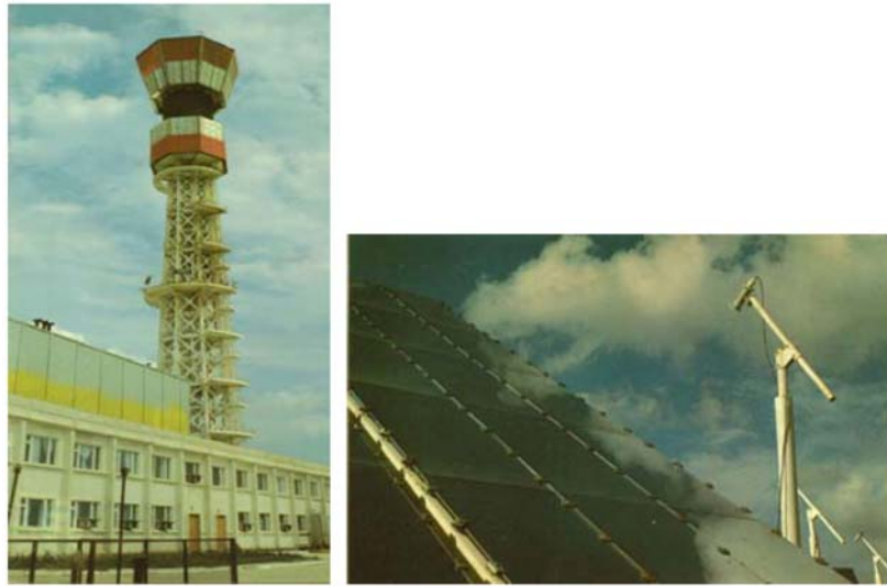
Figure 10. The tower of height 89m and optical probe for controlling the turn of heliostats in two planes are shown in photos; a number of heliostats is 1600, size 5 \times 5\text{m}^2 .
